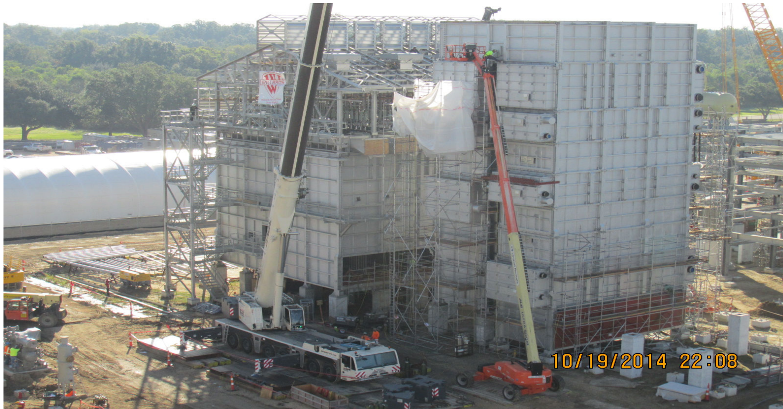
Reformer tube harps / spring hangers installed and roof sheeting installation
