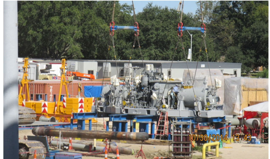
Synthesis gas compressor rigged for installation
