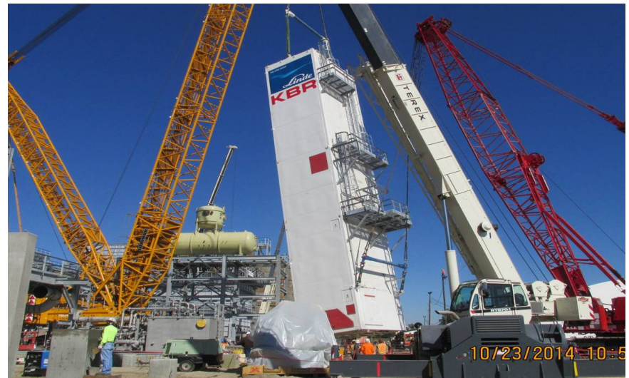
Ammonia tank refrigeration equipment under construction
