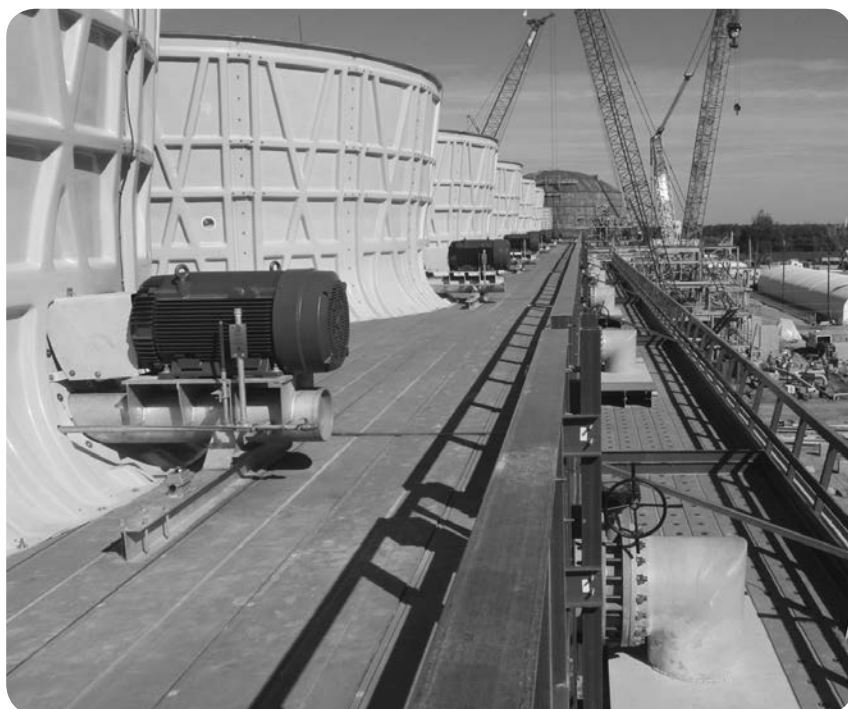
Cooling Tower and fan installation at Louisiana.
