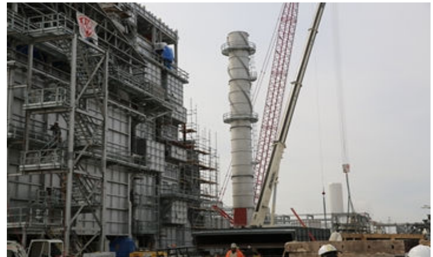
Secondary reformer crane pad being prepared
