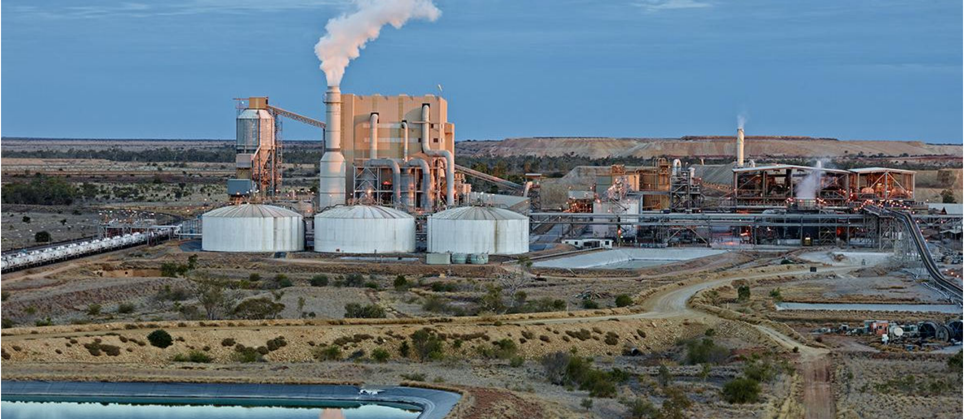
Picture: Phosphate Hill manufacturing facility, Qld, Australia
