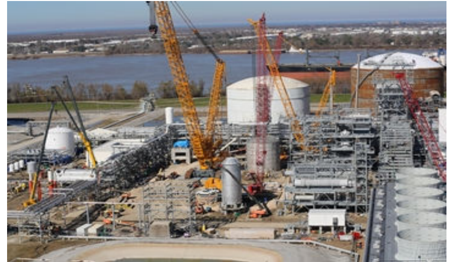
Overall construction view looking North
